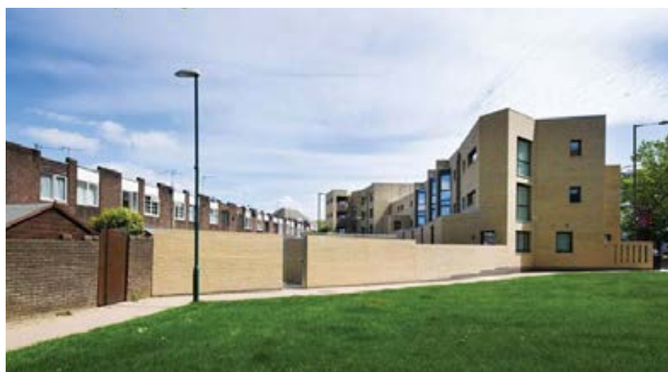
Grahame Park Phase 1B, new infill development defining the southern edge of the site
