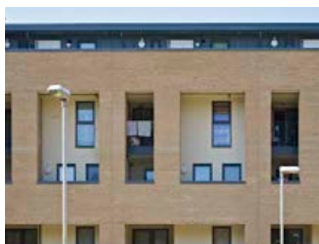
Concealed deck access, Hammond Court, Waltham Forest, London
