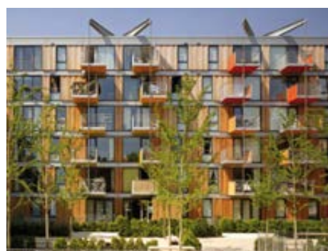
Prominent, lively frontage, Adelaide Wharf, Haggerston
