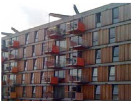
Prominent, lively frontage, Adelaide Wharf, Haggerston
