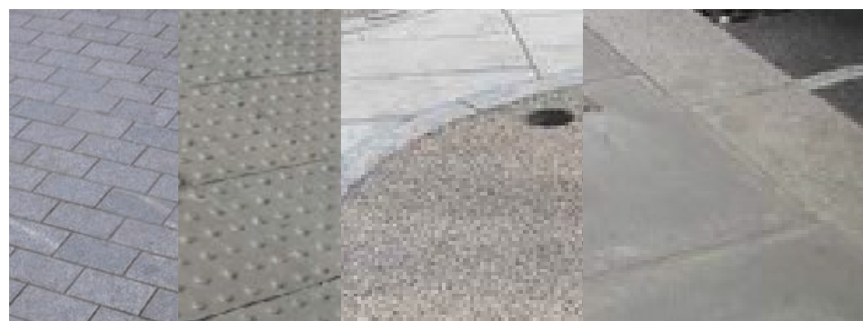
Granite setts for shared surfaces, grey blister paving, resin bound treepits, concrete pavers in public pathways and granite kerbs as edging create a normative palette to blend the estate into Colindale
