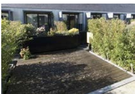
Raised garden decks above parking, with large voids and planting through, Chimney Pot Park
