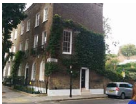
Articulated return on the building facade, Braes Street, Islington
