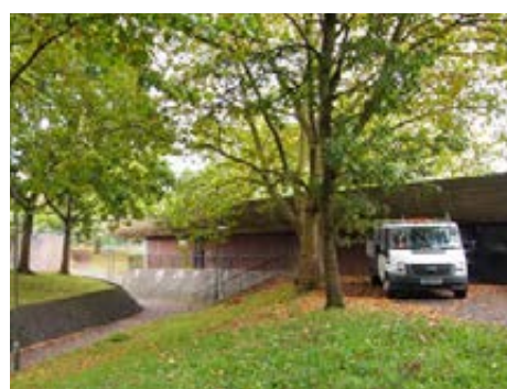
Existing energy centre
