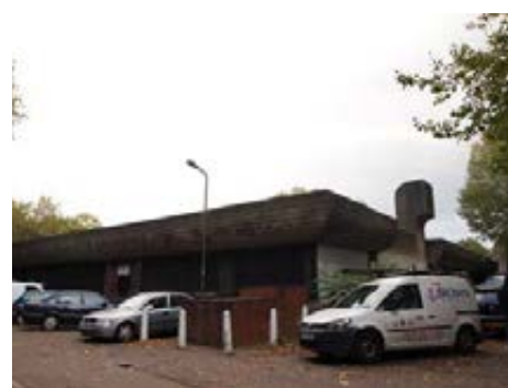
Existing energy centre
