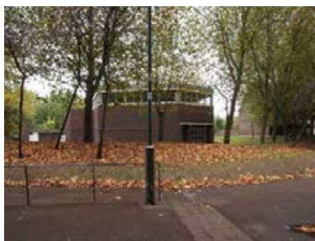
The existing church
