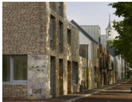
Informal building heights, Molenplien, Netherlands
