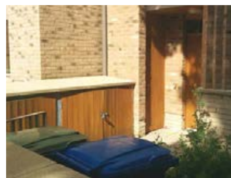
Integrated storage and bins area by dwelling entrance, Royal Road, London
