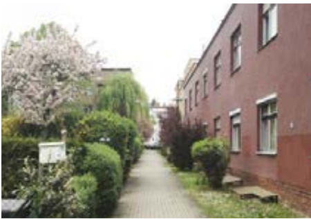
Frontages facing private rear gardens, with permeable boundary treatments and planting, Britz Metropolitan, Berlin
