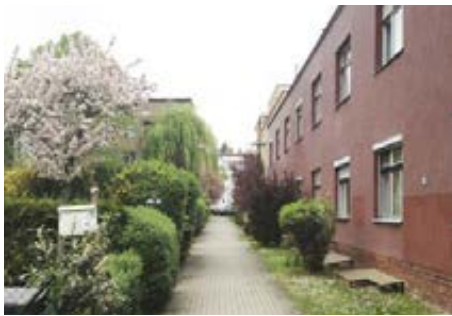
Frontages facing private rear gardens, with permeable boundary treatments and planting, Britz Metropolitan, Berlin
